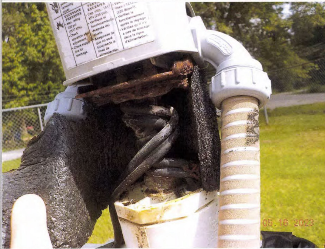
Documentation of the flow switch for the well meter with significant rust.
