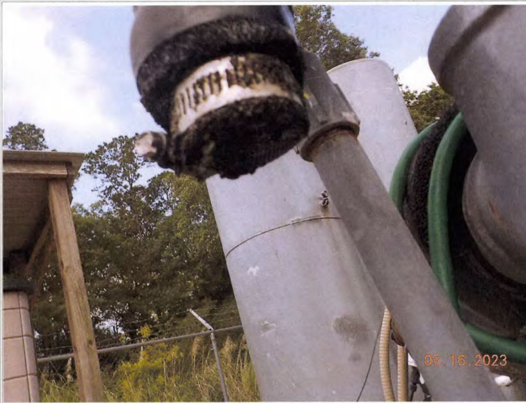
Documentation of the 16-mesh screen on the well vent with mold.
