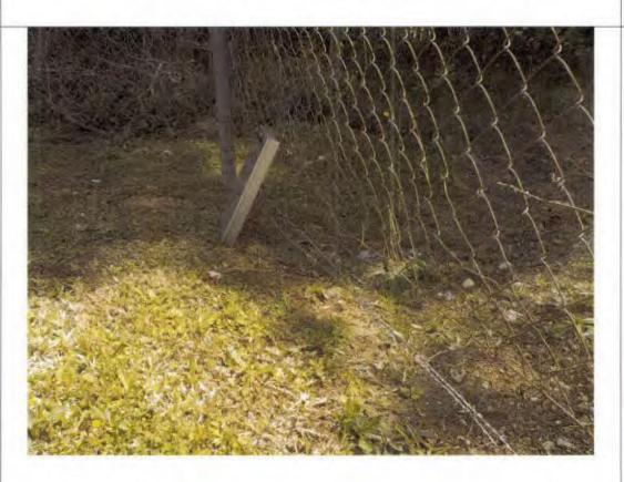
Photograph documenting the large gap under the backright side of the water treatment plant's fence that were loose enough that the bottom could be pulled upward and potentially allow entry into the water treatment plant. Please note that there were two strands of barbed wire blocking the gaps under the left side of the fence.
