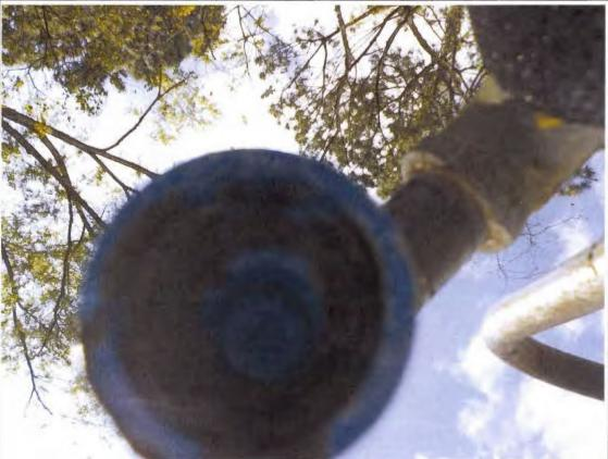
Photograph documenting the second air release device on Well No. 1 that did not have its opening covered with 16-mesh corrosion-resistant screening material.
