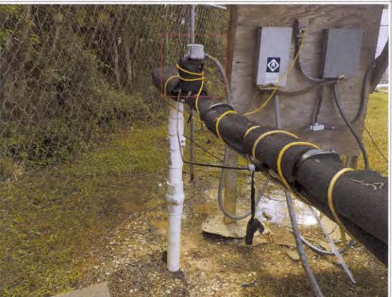
Photograph documenting the wiring for Well No. 1's pressure switch, which was detached from the pressure switch's housing. Because of this, the pressure switch's electrical wiring was exposed.
