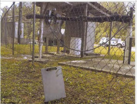
Photograph documenting the large gap under the left-back side of the water treatment plant's fence that were loose enough that the bottom could be pulled upward and potentially allow entry into the water treatment plant. Please note that there was one strand of barbed wire blocking the gaps under the back side of the fence.
