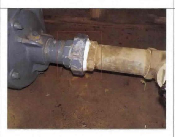
Photograph documenting the leak on the inlet waterline for the blue service pump at Plant No. 1.
