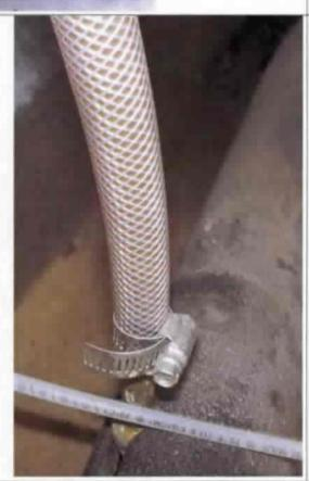
Photograph documenting the top (left) and bottom (right) ends of the clear hose that was being used as a sight glass for the 900-Gallon Pressure Tank at Plant No. 2.
