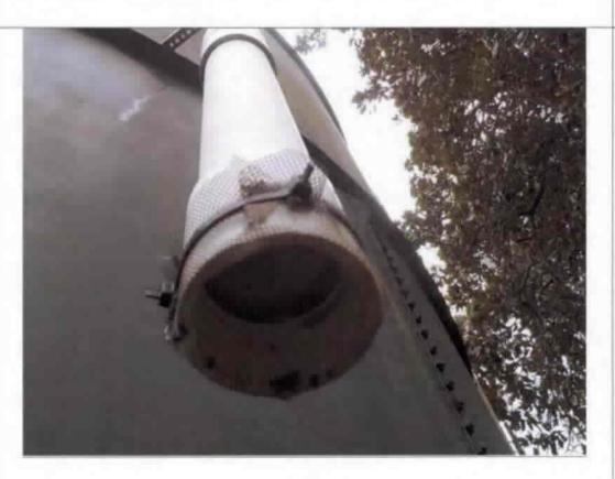
Photograph documenting the 16-mesh screening material that covered the end of the overflow pipe for the Green 0.022 MG ground Storage Tank at Plant No. 1. Please note that there was no gravity-hinged and weighted cover, an elastomeric duckbill valve, or other approved device equipped on this tank's overflow pipe.
