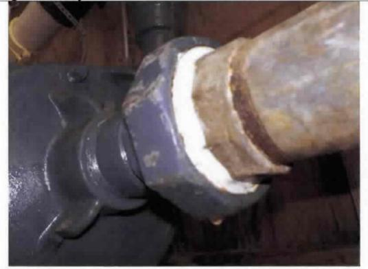
Photograph documenting the leak on the inlet waterline for the blue service
