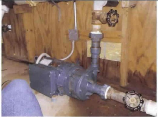
Photograph documenting the leaks on the inlet and outlet
