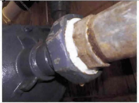
Photograph documenting the leak on the inlet waterline for the blue service pump at Plant No. 1.
