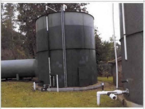
Photograph documenting the lack of a liquid level indicator on the Green 0.022 MG Ground Storage Tank. Please note that there was a liquid level indicator on the Galvanized 0.022 MG Ground Storage Tank.
