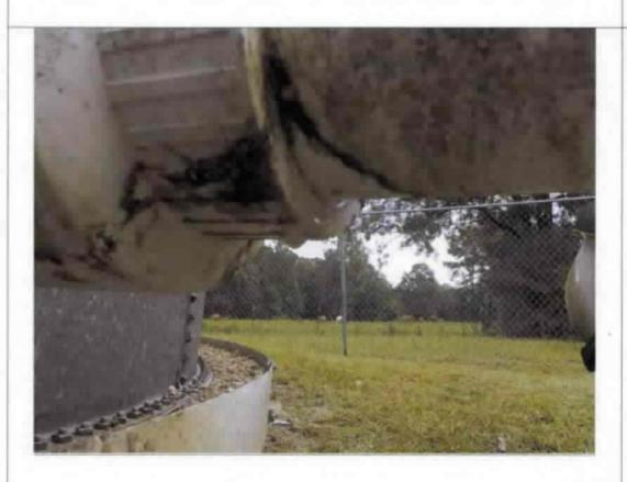
Photograph documenting the leak on the outlet pipe to the Galvanized 0.022 MG Ground Storage Tank at Plant No. 1.
