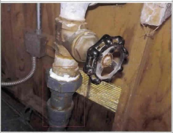
Photograph documenting the leaks on the outlet waterline for the blue service pump at Plant No. 1.
