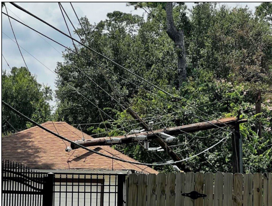
Figure RP-7 Broken poles from tree falling
