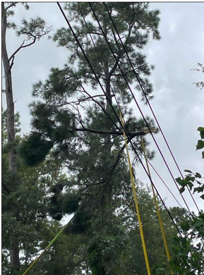
Figure RP-6 Treetop falling into power lines
