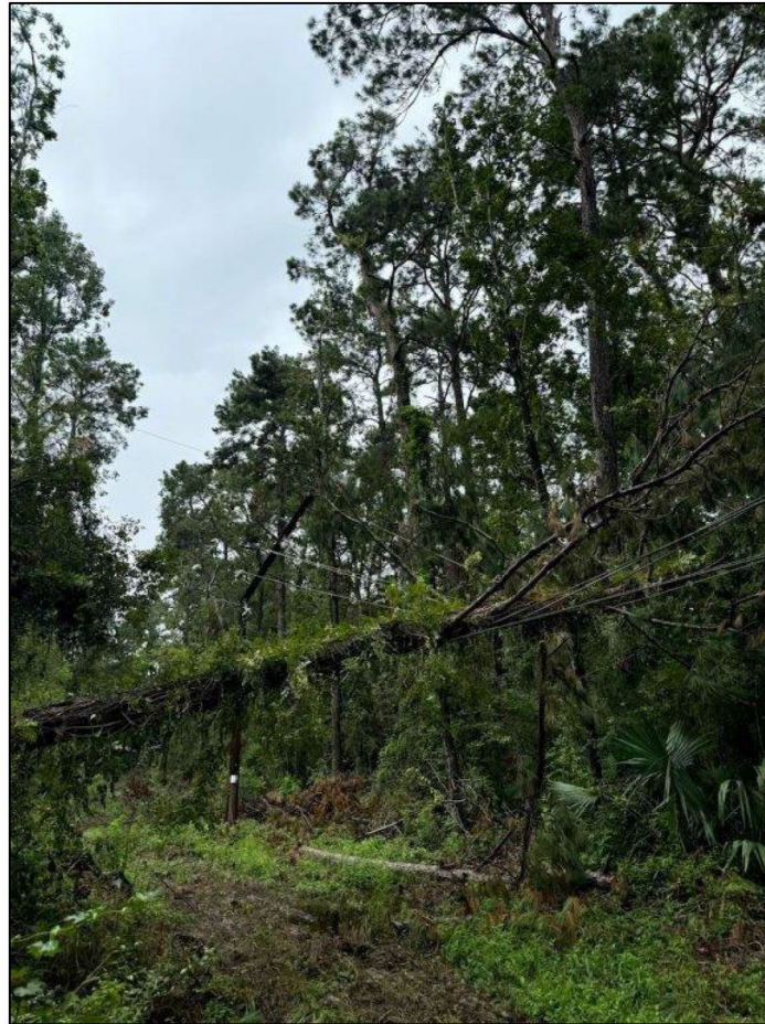
Figure RP-5 Tree outside of easement causing outage
