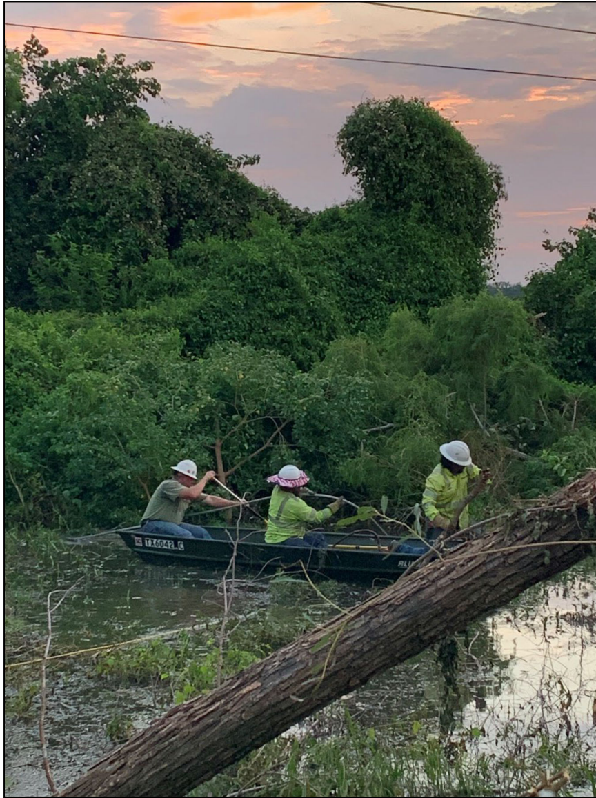
Figure RP-8 Fallen conductor in water
