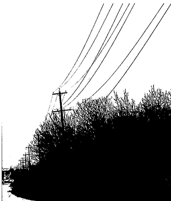
Figure 3-6. Tree-caused Outages Branch Burn Off. New growth has been "burnt off" from occasional line contact.
