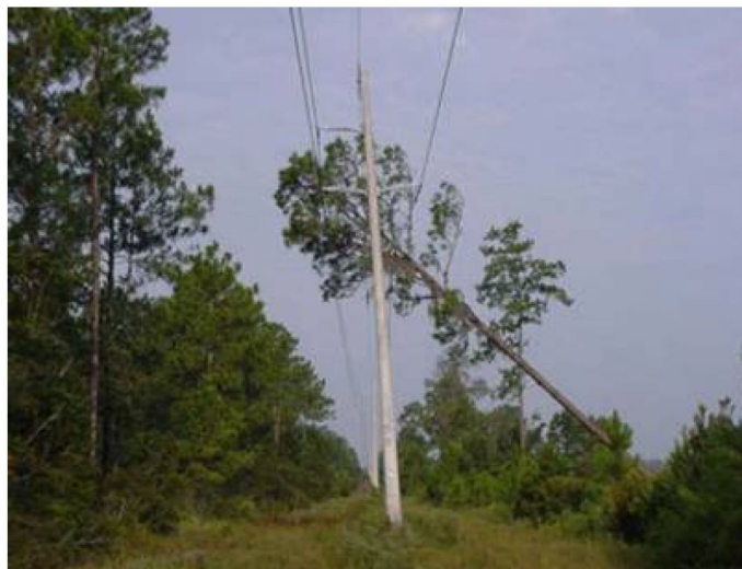
Figure 2-1. A danger tree is a tree that is tall enough to fall into nearby power lines.
