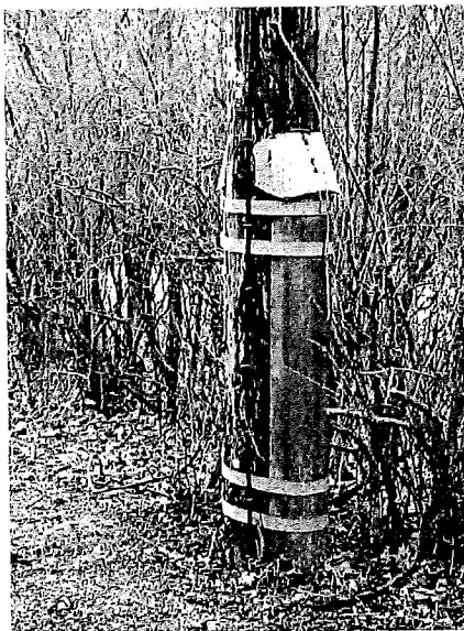
Figure 14. C-Truss Pole Reinforcement (Rockford)
