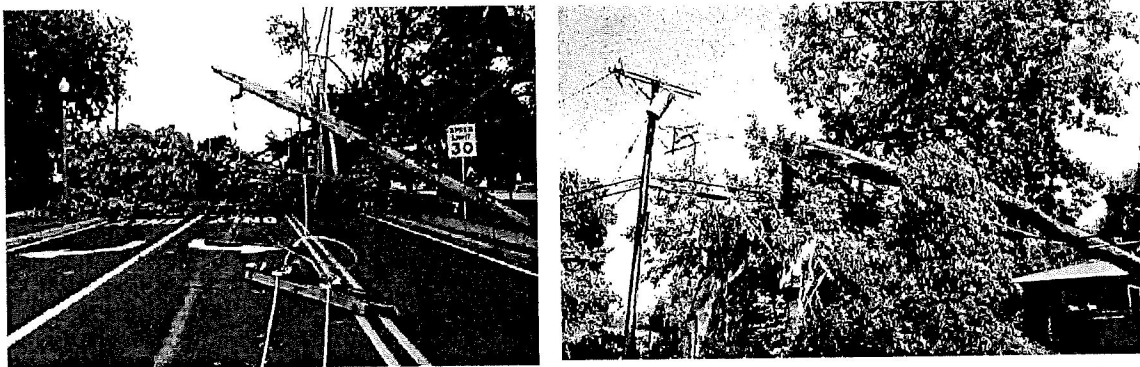
Figure 3. Example Storm Damage from Uprooted Tress
