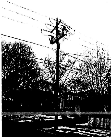
Figure 8. Intelli-Rupter on 12.47 kV Line (Rolling Meadows)
