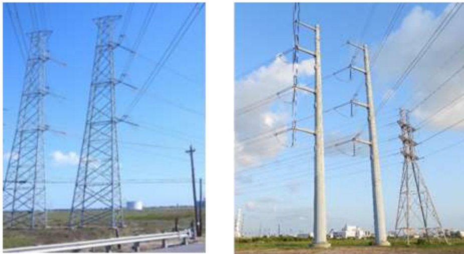
Figure 5-5: Typical Transmission Towers Before and After Replacement
