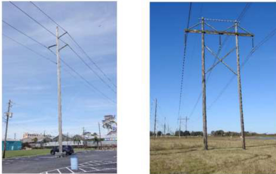
Figure 5-4: Examples of Transmission 138kV Wood Structures
