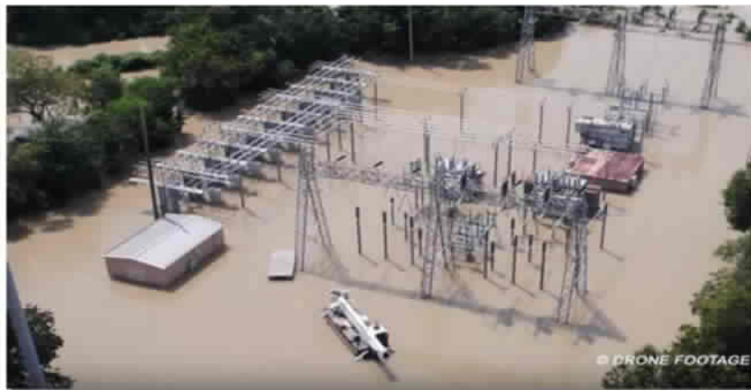
Figure DM-7 Flooding to a Company Substation
