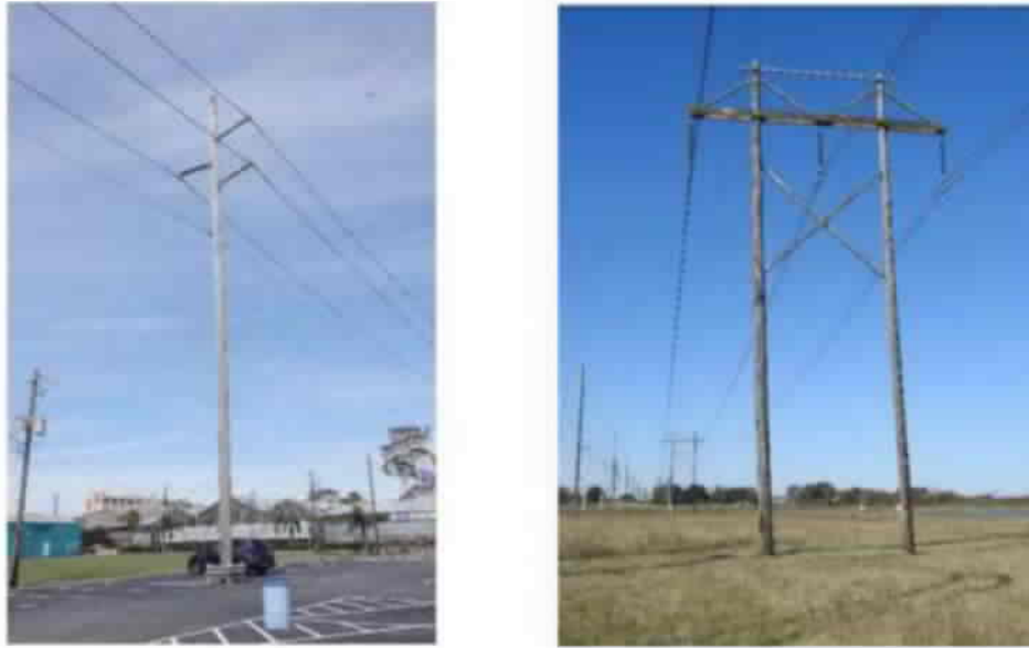
Figure 5-4: Examples of Transmission 138kV Wood Structures
