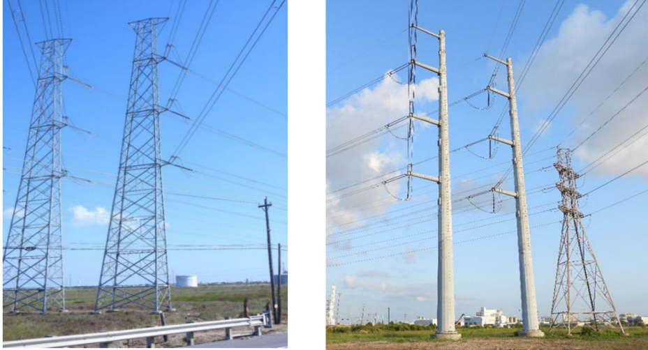
Figure 5-2: Typical Transmission Towers Before and After Replacement
