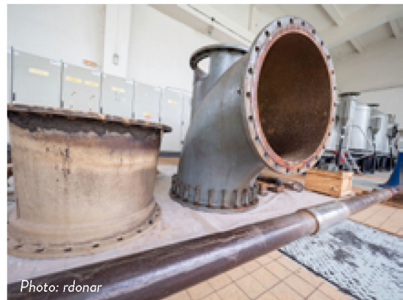
AXIAL HYDRODYNAMIC FLOW PUMP IN WASTEWATER PLANT.
