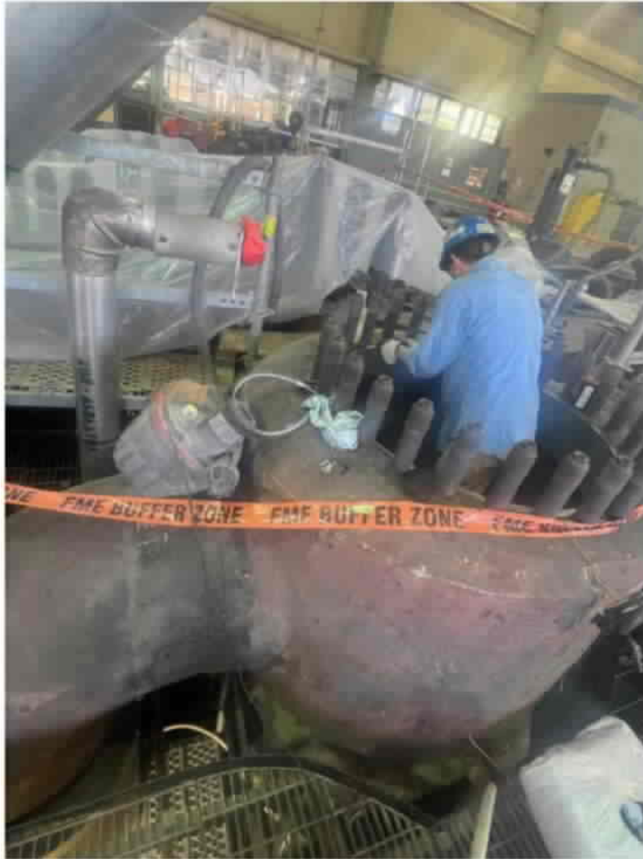
Cleaning Turbine Valve Gasket Surfaces
