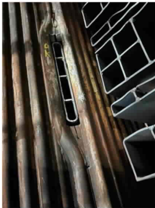
Natural Gas Burners on Boiler Corners
