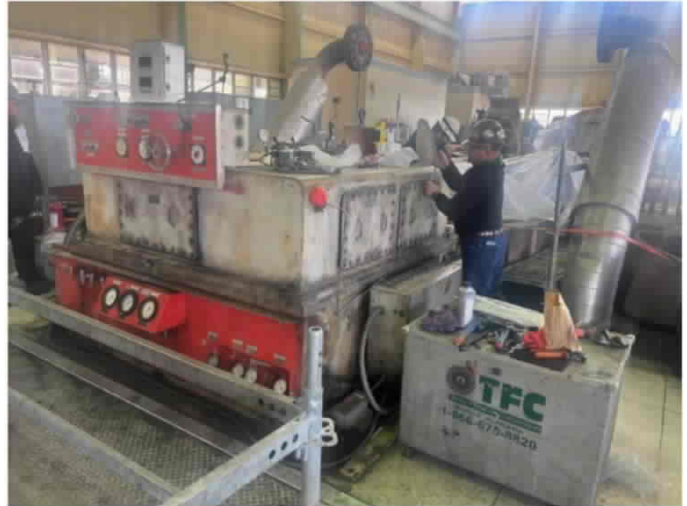
Turbine front standard covers installed for lube oil flushing
