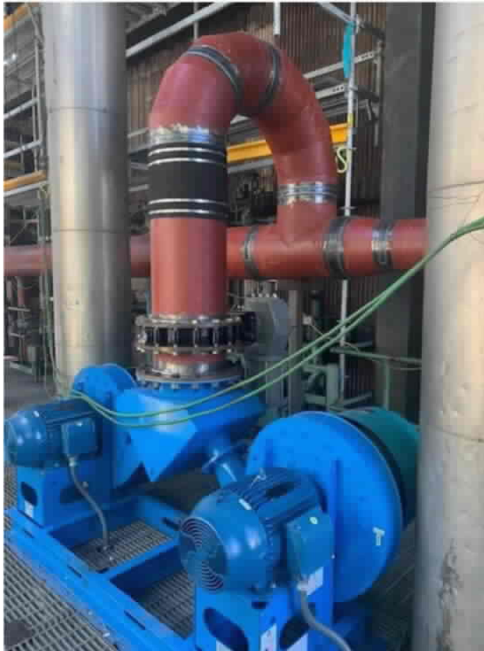
Ignitor Scanner Air Fans and Piping
