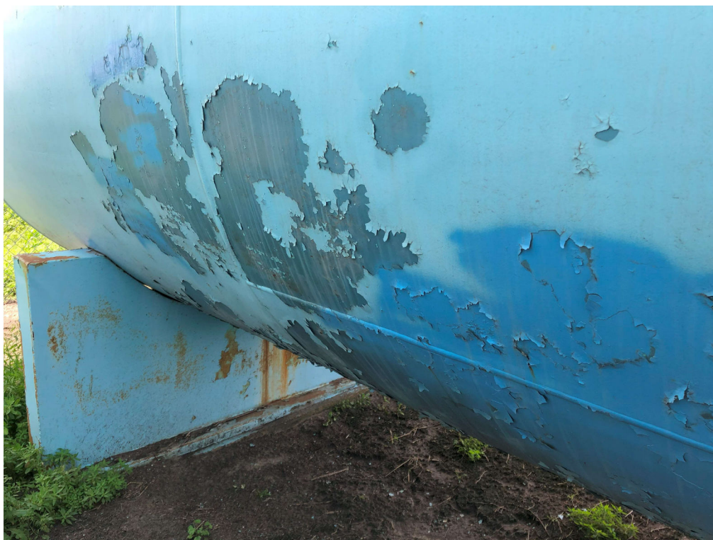
Photo #23: Coating conditions on 5,000-gallon Hydropneumatic Tank
