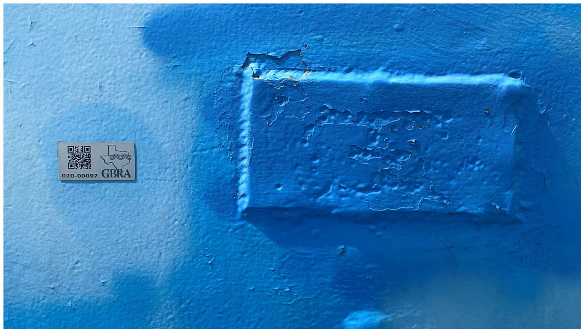
Photo #24: Missing Label on 5,000-gallon Hydropneumatic tank
