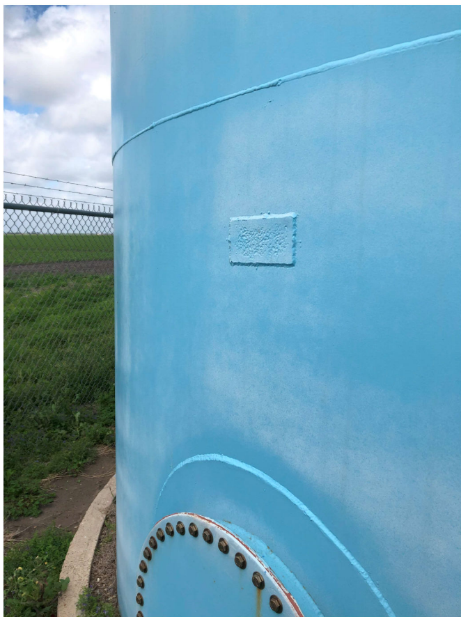
Photo #18: Missing Tank Label on 34,000-gallon Ground Storage Tank
