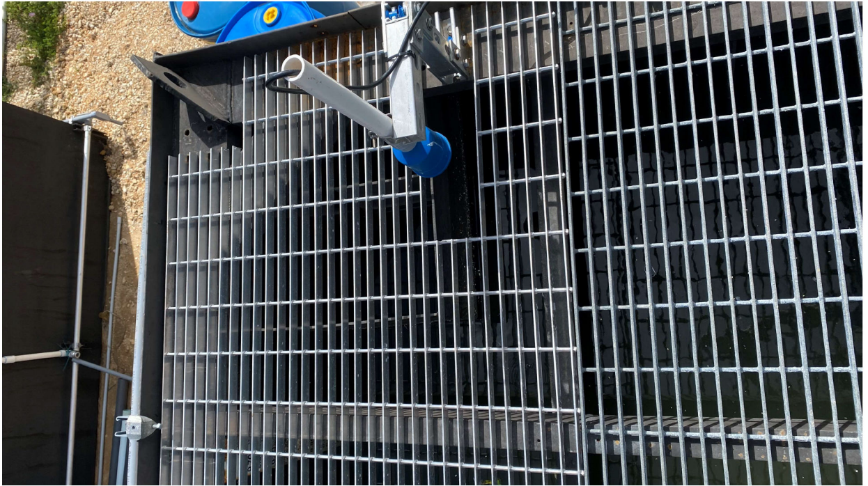
Photo #13: Effluent Flow Measuring Device
