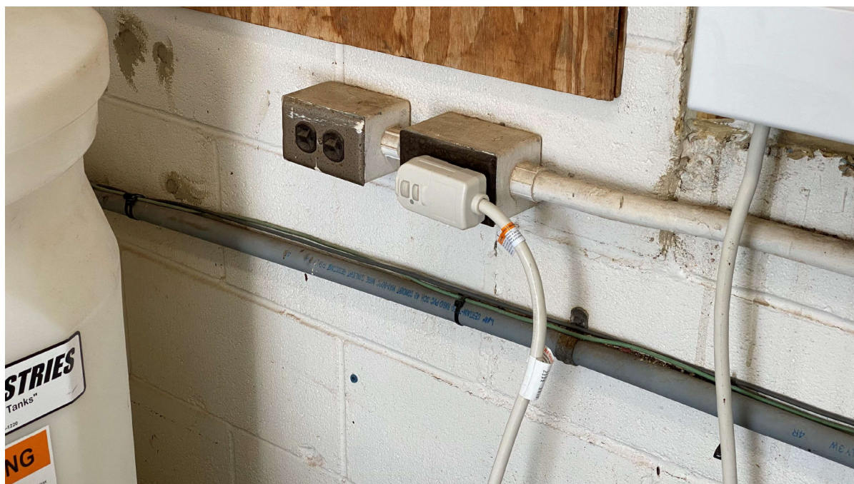
Photo #20 Electrical outlets inside Booster Pump Station
