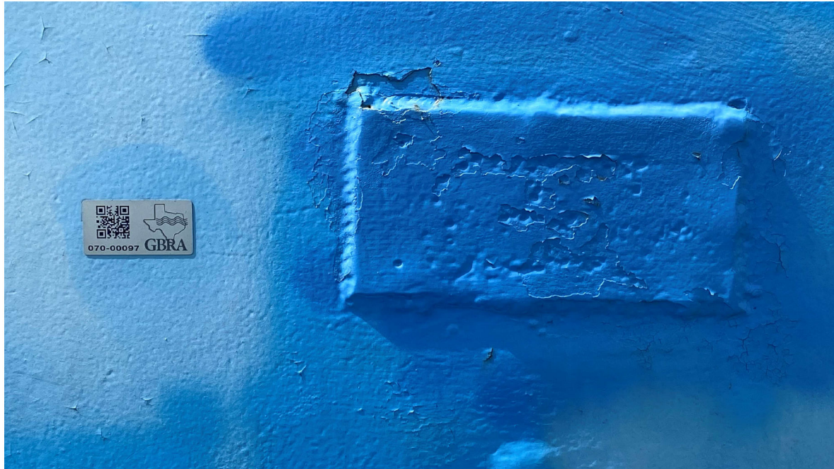
Photo #24 Missing Label on 5,000-gallon Hydropneumatic tank
