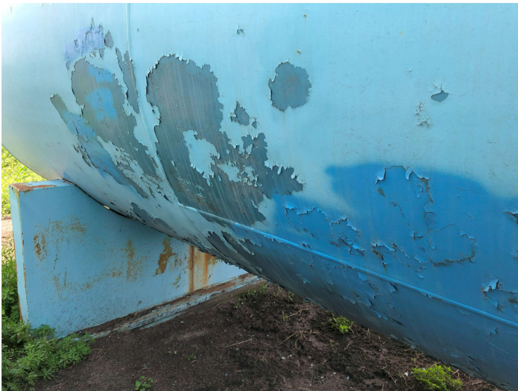
Photo #23 Coating conditions on 5,000-gallon Hydropneumatic Tank
