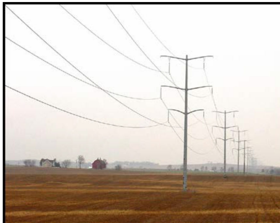
Figure 2 Typical Single-Pole, Double-Circuit Structure
