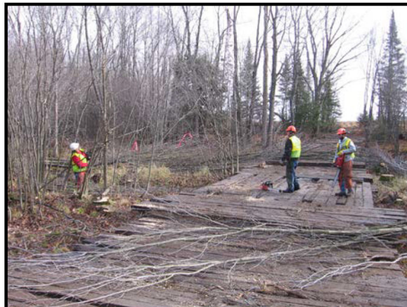
Figure 10 Hand Clearing Channel
