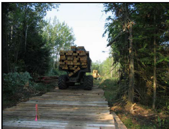
Figure 8 Mats Used in a Wooded Wetland
