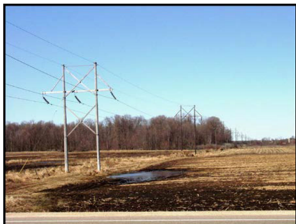
Figure 1 Typical Two-Pole, H-frame Structure
