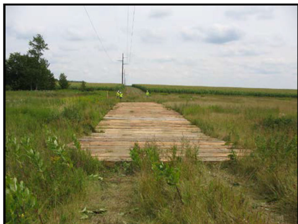
Figure 7 Mats Used in a Wet Meadow
