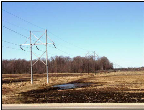
Figure 1 Typical Two-Pole, H-frame Structure
