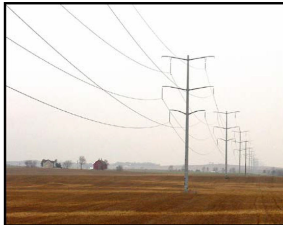
Figure 2 Typical Single-Pole, Double-Circuit Structure
