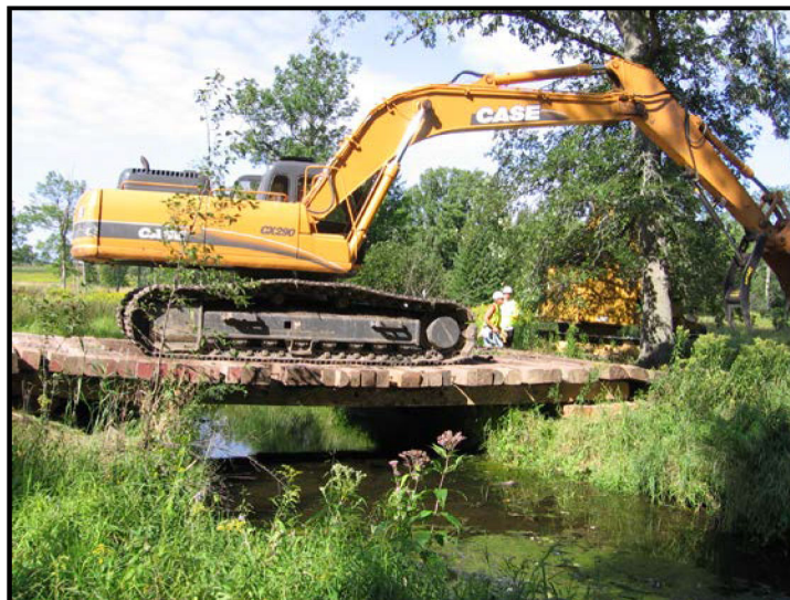
Figure 5 Temporary Bridge Structure Spanning a Waterway
