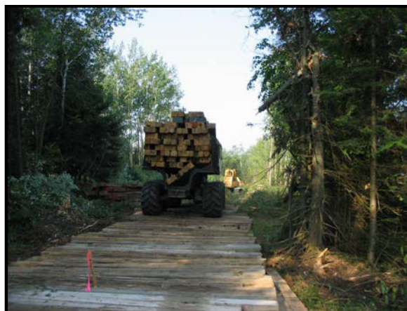
Figure 8 Mats Used in a Wooded Wetland
