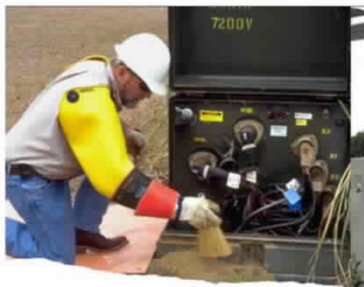
Figure 6 – Padmount Transformer
