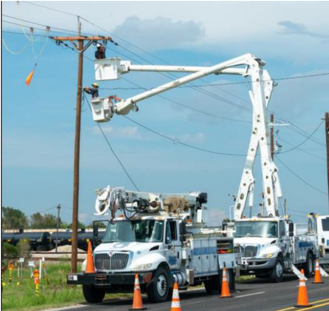
Figure 2 - Crew replacing a broken cross-arm and cross-arm braces
