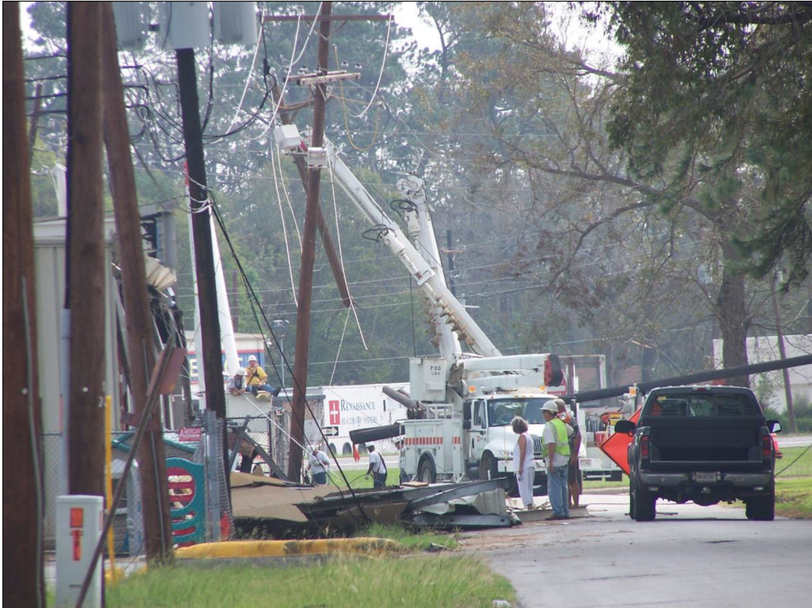
Figure 1 - Crew replacing a broken pole
