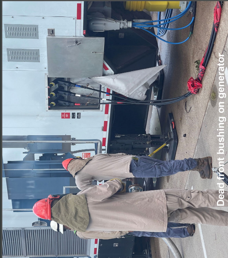
Connection on High-side of Customer's transformer Used Standard Terminators to connect to the Fuse cutouts.
