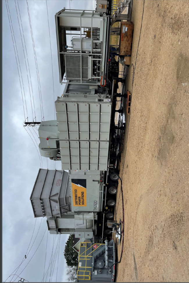
GE TM2500 Gen 8 ~32MW Liquid Fuel or Natural Gas 12.47kV
