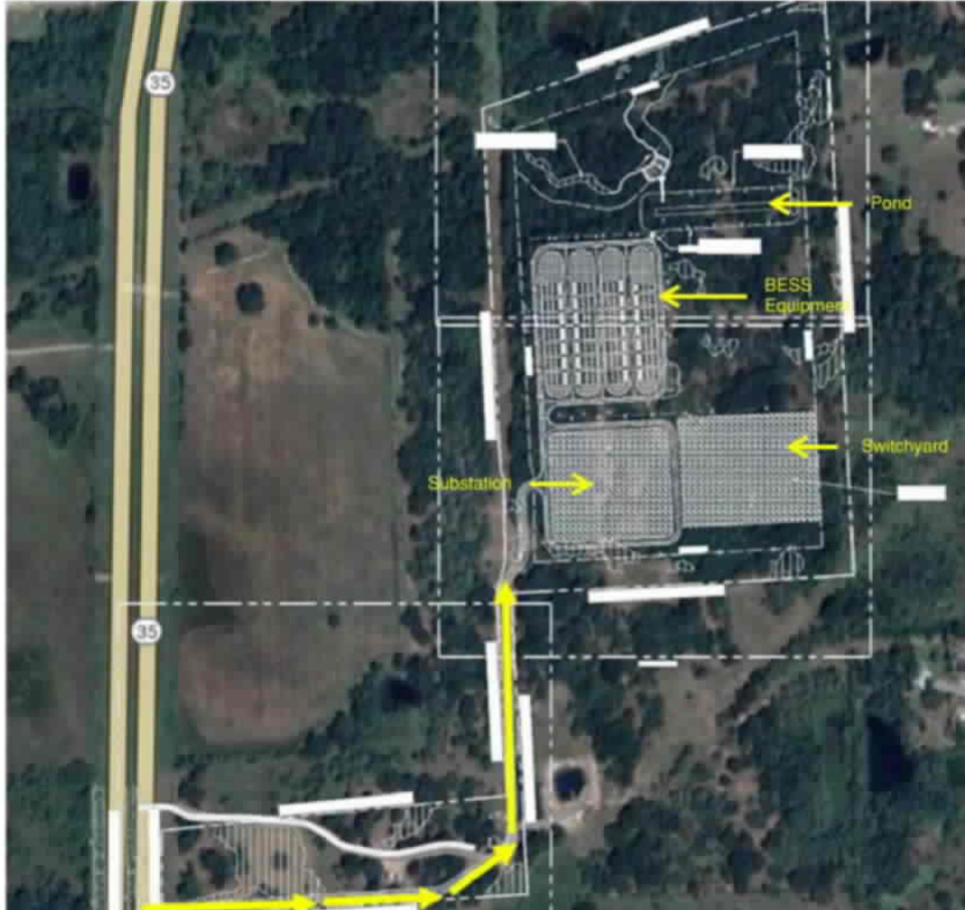
Figure 3-3: Aerial Overview of Bell Creek BESS
