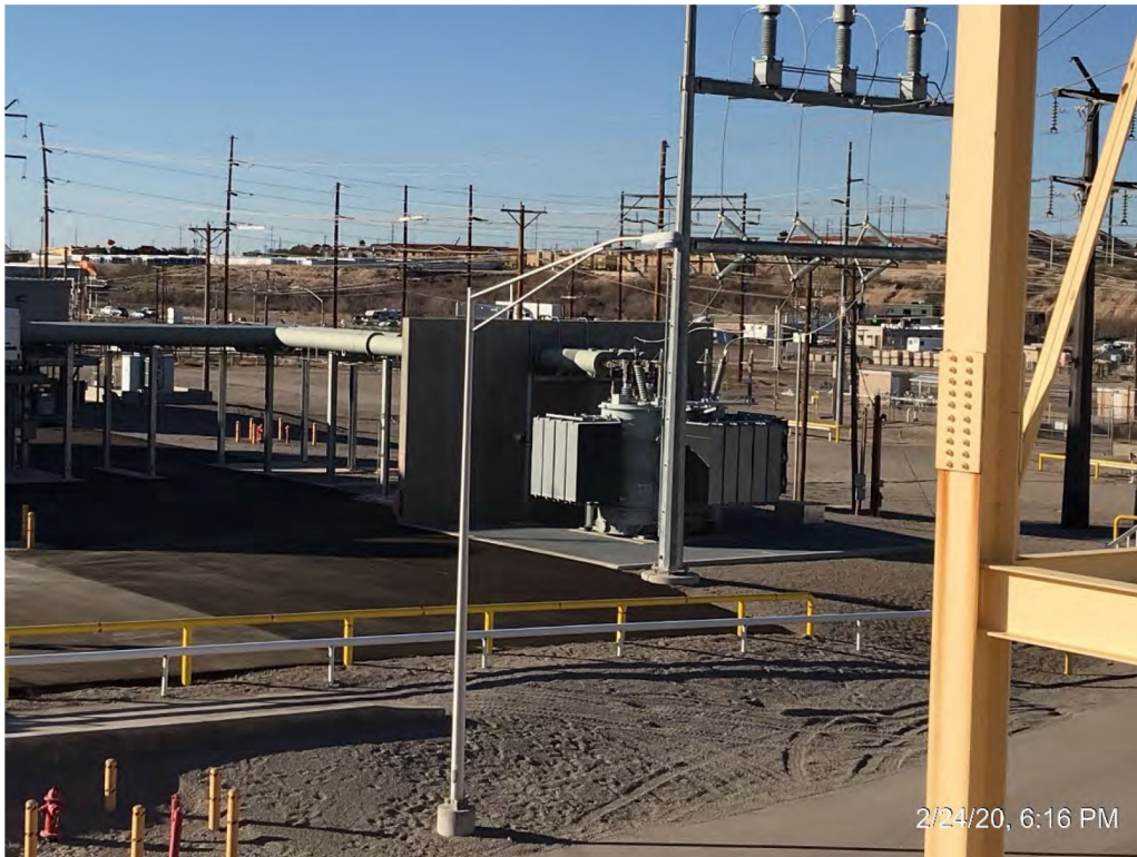
Account 346, Miscellaneous Power Plant Equipment Unit 9 GSU
