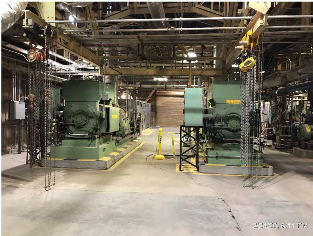
Account 312, Boiler Plant Equipment Unit 8 Boiler Feed Pumps
