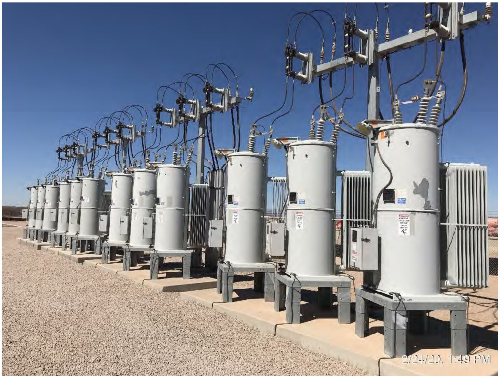
Account 353, Station Equipment Regulators
