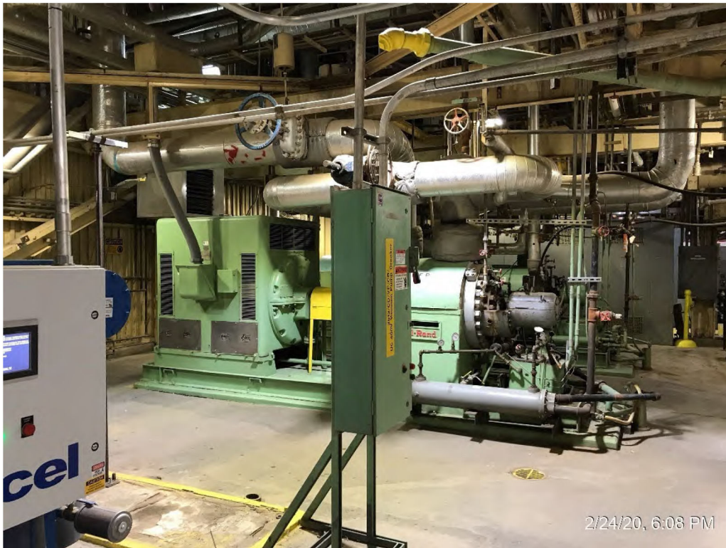
Account 312, Boiler Plant Equipment Unit 6 Boiler Feed Pump
