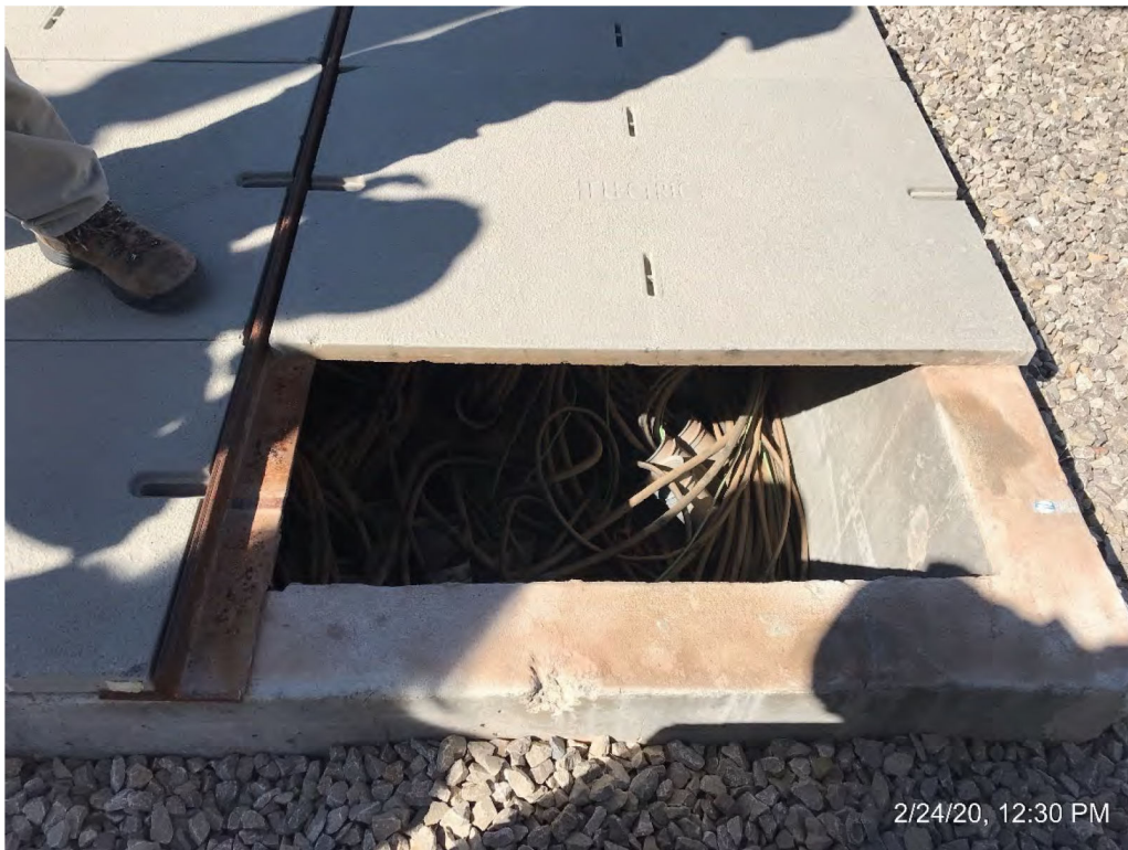
Account 353, Station Equipment Pull Box at Substation
