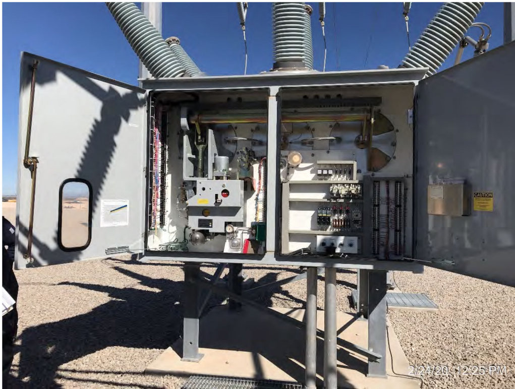
Account 353, Station Equipment Interior of Breaker at Substation
