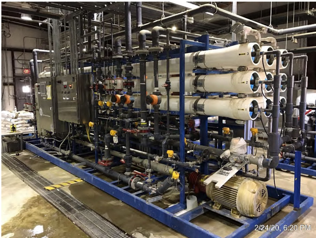
Account 346, Miscellaneous Power Plant Equipment Reverse Osmosis System
