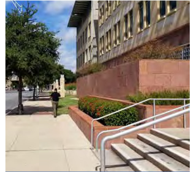
South entrance to the Durango Building
