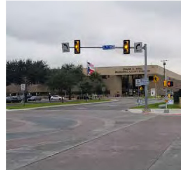
Frank D. Wing Municipal Court Building
