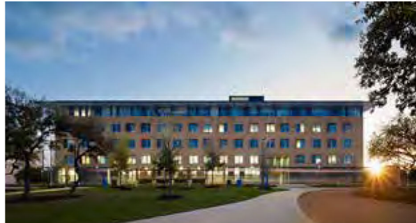
North Paseo Building
