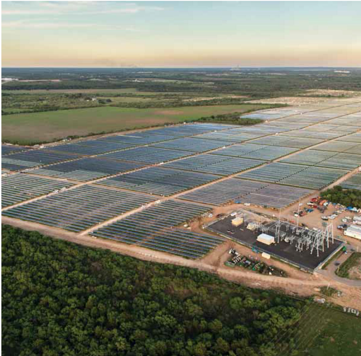
Investment in renewable energy sources, such as the Blue Wing Solar Project, are vital and will create a more resilient and sustainable San Antonio.
