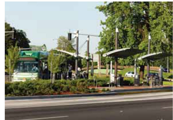
The EMX bus rapid transit system connects several neighborhoods, employment centers, a new hospital and mixed-use districts in Eugene and Springfield, Oregon.
