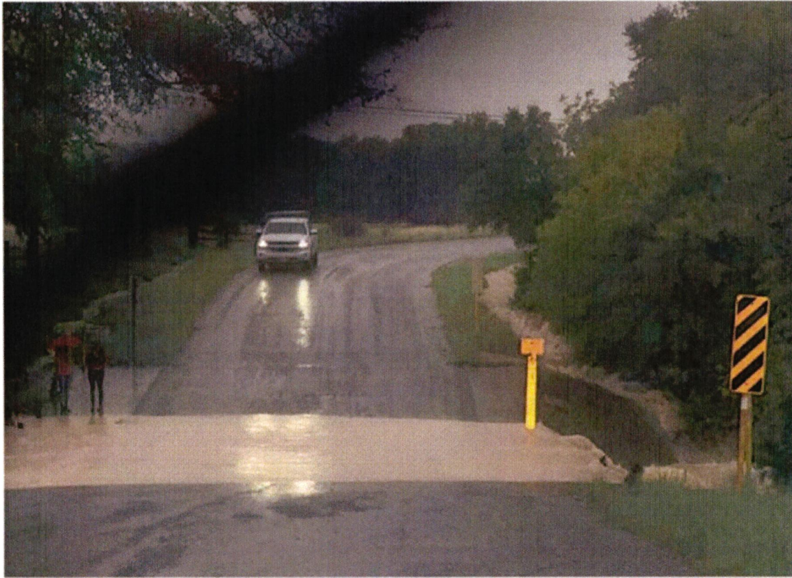
A Huntress lane low water crossing with flooding (9/2018)
