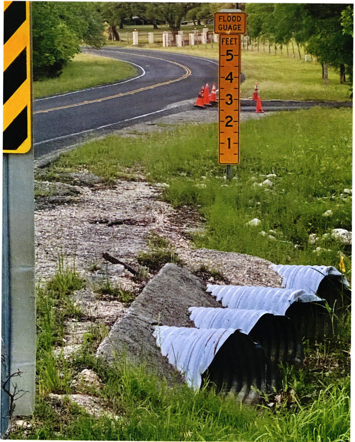
Flood gauge near entrance to Anaqua Springs Ranch subdivision.
