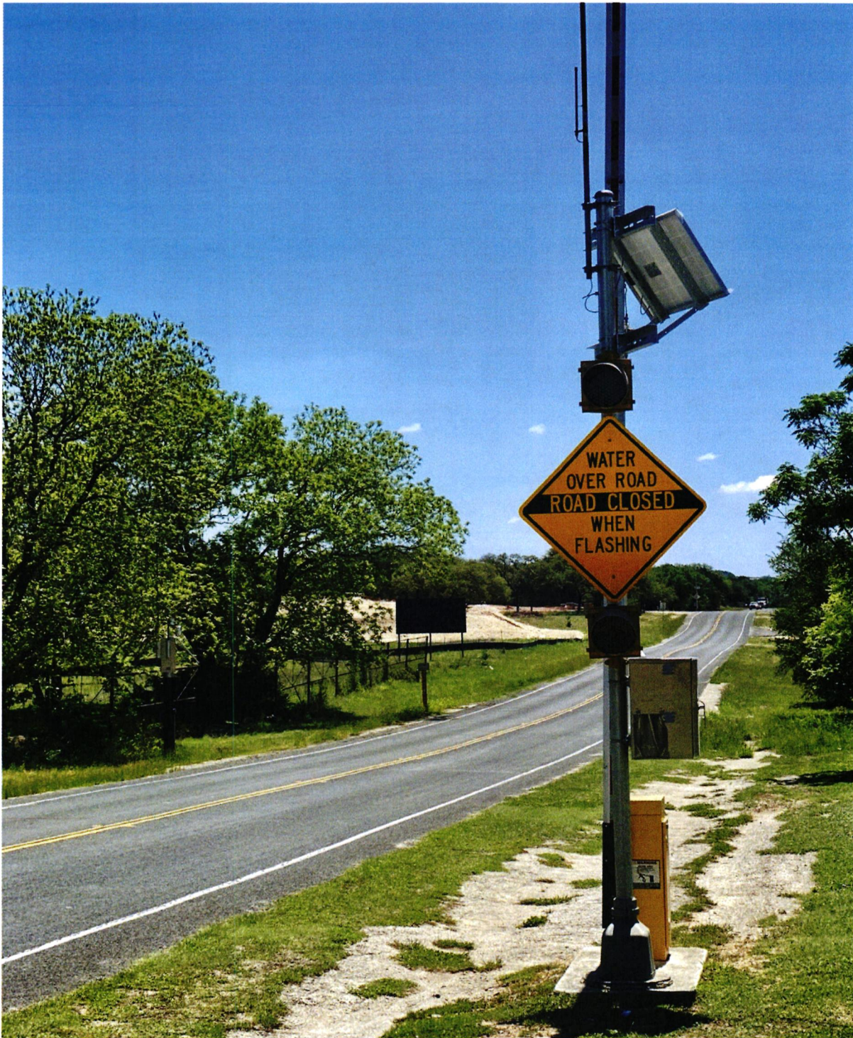
One of four flood gates/warning signals located on Toutant Beauregard Road between Sundance Ranch subdivision and McAndrews Elementary School. This one is located near the entrance to Sundance Ranch subdivision.
