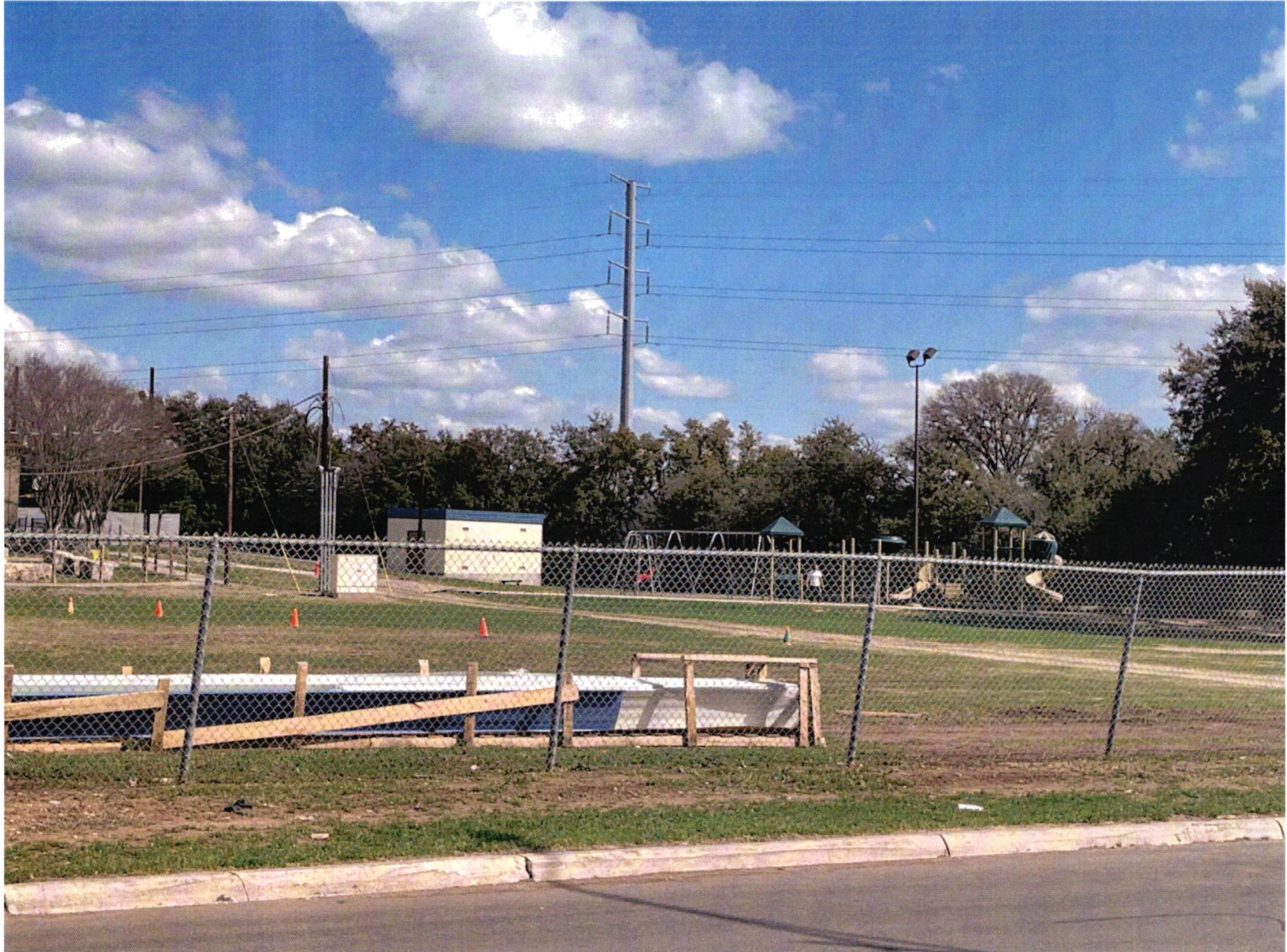
Elrod Elementary School - NISD - March 8, 2021
