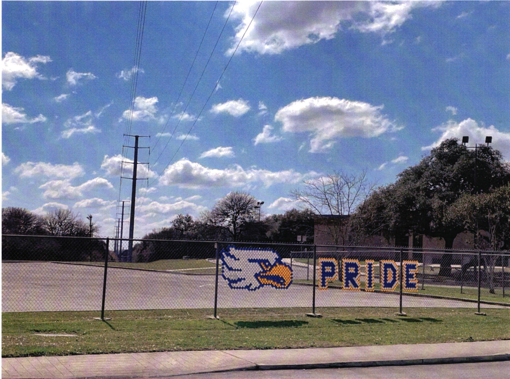
Elrod Elementary School - NISD - March 8, 2021
