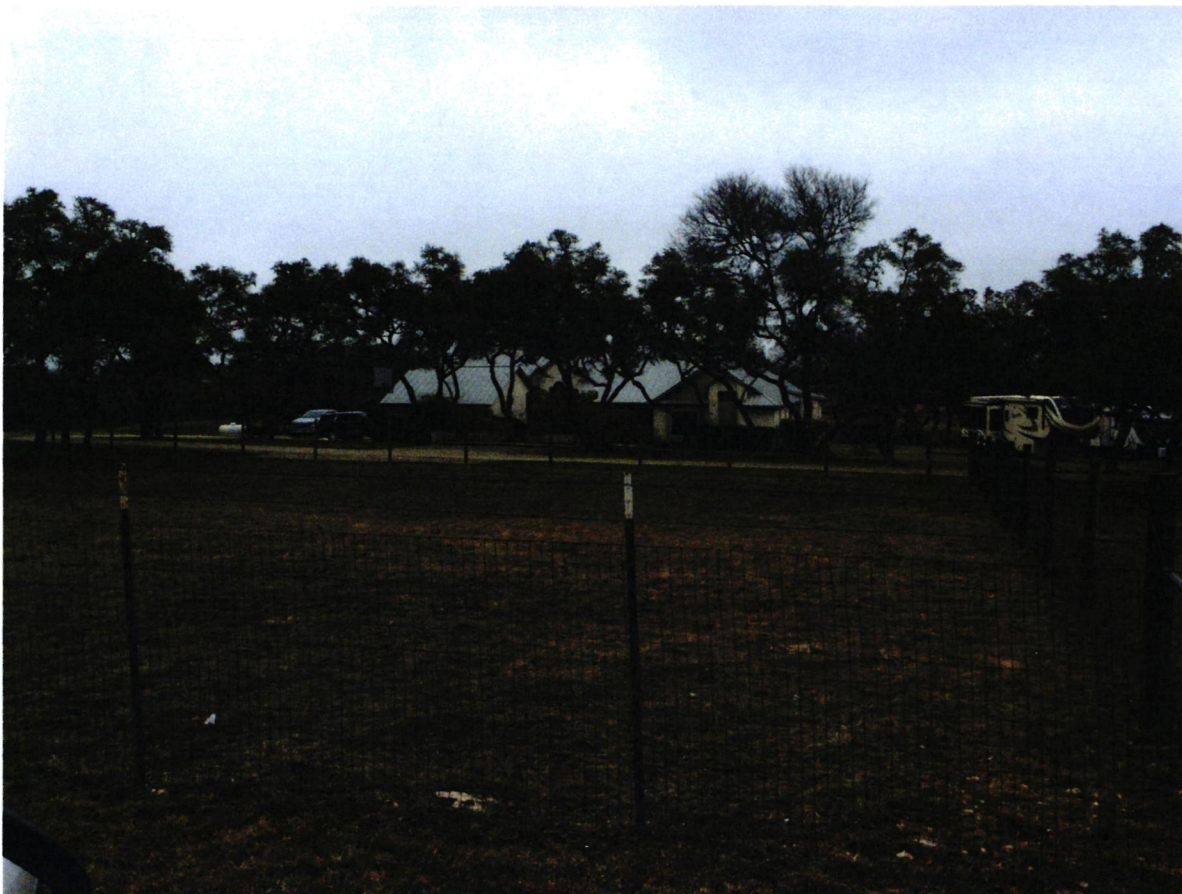
Habitable structure No. 78, adjacent to Substation Site 7.
