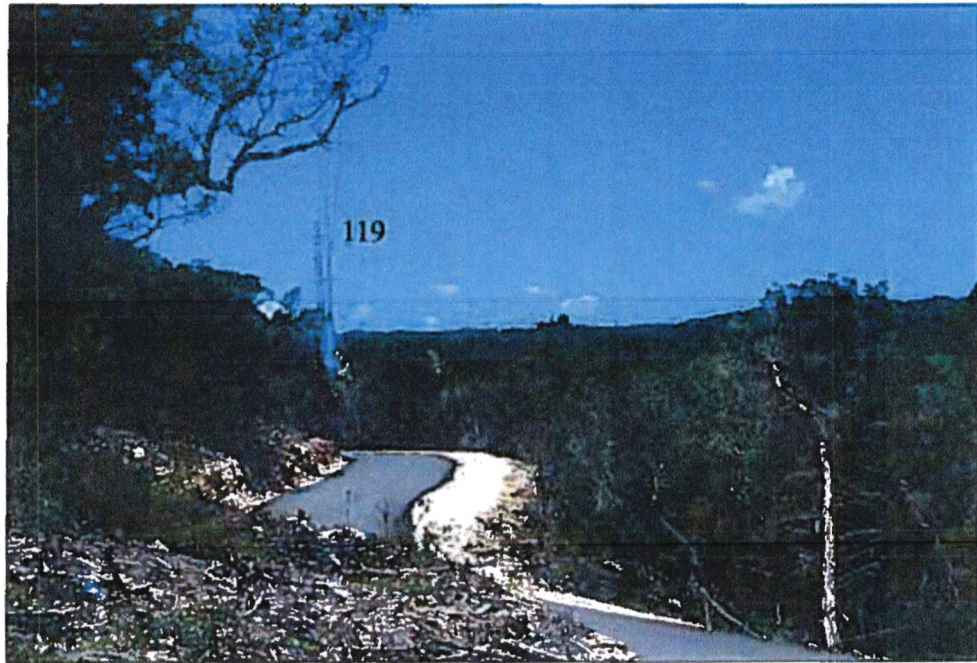
Photograph 6 - Area 3. Looking west from Pole 120 along the permanent access road toward Pole 119.
