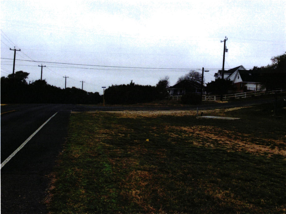
North side of Toutant looking west to the intersection of Lost and Toutant. Habitable structures 88 and 89 are visible on the right side of photo. Segment 54 crosses Toutant directly in front of No. 88, which is the white house on the corner.
