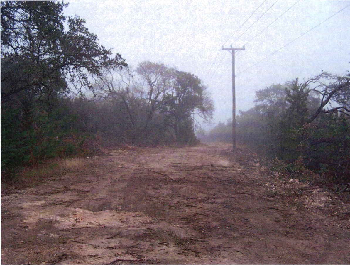
Looking to the east on the back of my property showing where CPS deviated from its easement into my property, clearcutting my land
