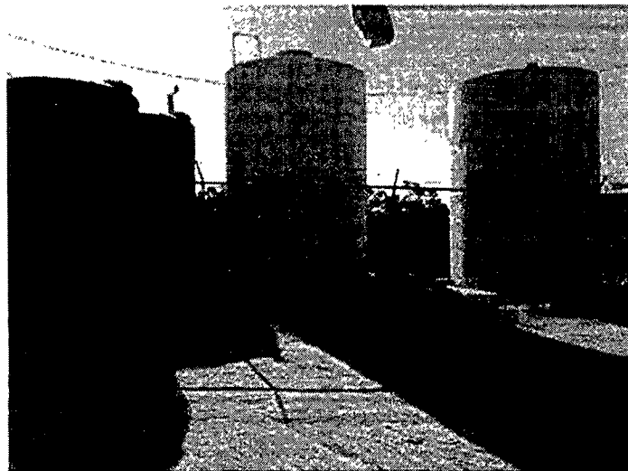
11. Vinton Village welded steel tanks and on site poly replacement tanks
