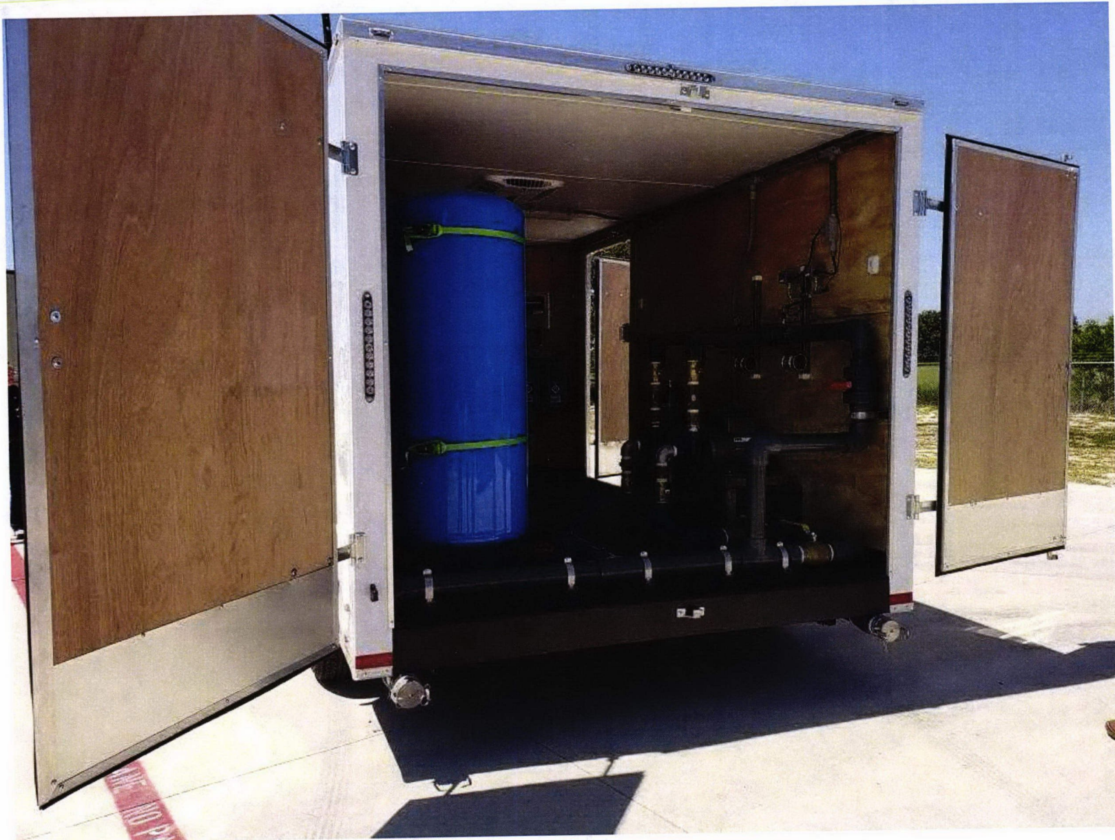
Mobile Pump House Trailer
