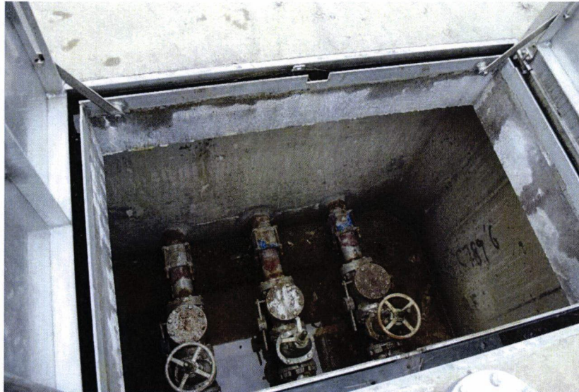
Figure 12-6: Valve Boxes at Carter Ranch LS
