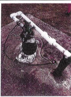
Photograph 4 shows the wellhead on Well 3 improperly sealed, and electrical wiring without conduit.
