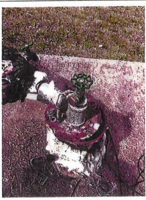
Photograph 2 shows the well vent screen detached from Well 1.
