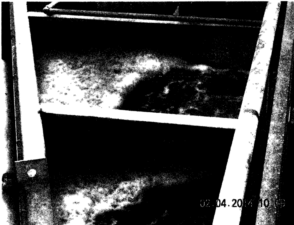
This is a photo of the chlorine contact basin. Notice the foam and scum in the basin.
