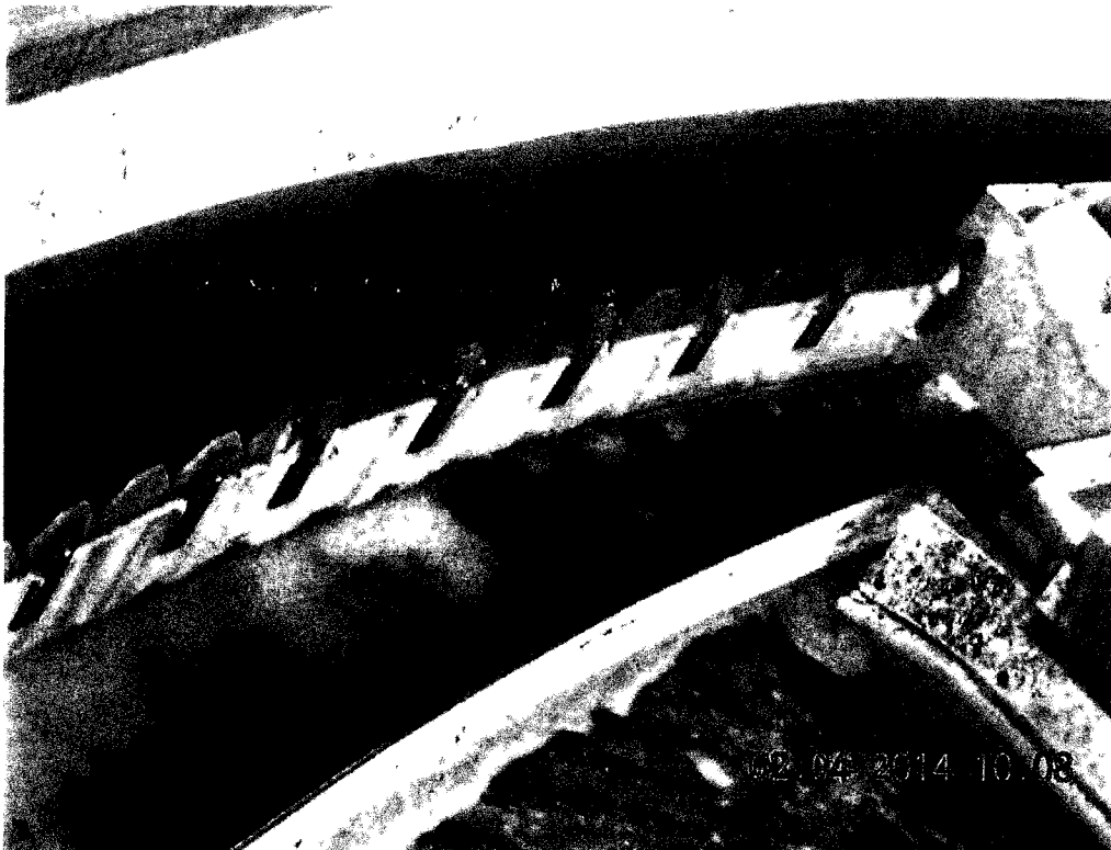
This is a photo of the clarifier. Notice that there is no flow over the weirs on this section of the clarifier.
