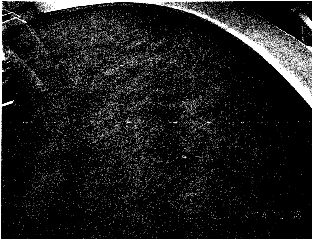
This is a photo of the aeration basin overwhelmed with foam at the time of the investigation.
