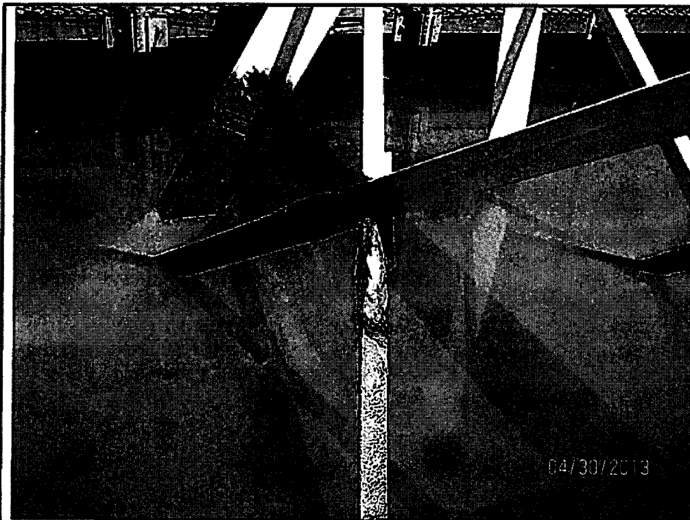
Picture #1 – At the time of the investigation, there was significant rust along the flocculator arms at the North Water Treatment Plant.
