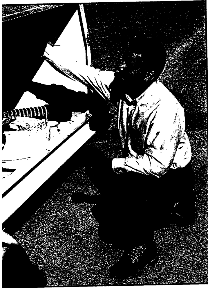
Rural Utilities Manager Mike Urrutia inspects a jetting machine that is used to clean out sewer lines.
