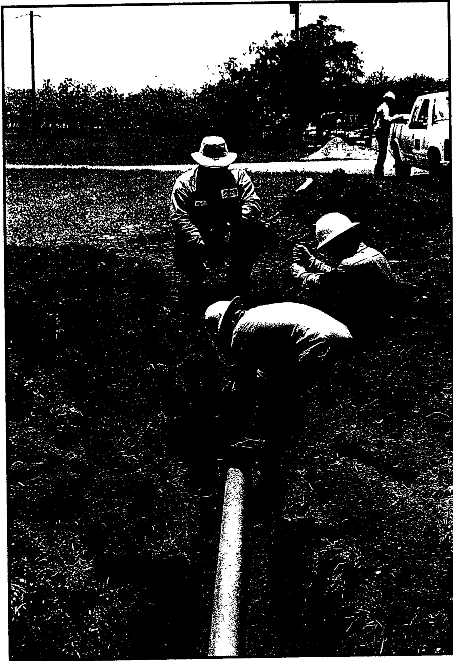
Ron Gosnell, Chief Operator; Don Koble, Senior Operator; and Ryan Boedeker, Maintenance Operator relocate water lines at the intersection of FM 1090 and Royal Road due to a state highway expansion project.
