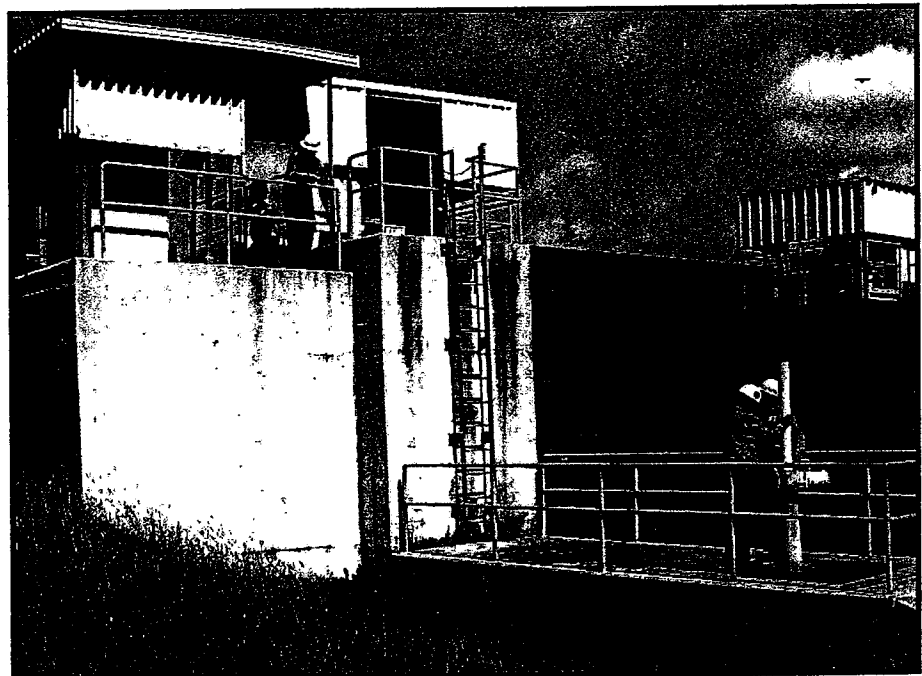
Coletto Reservoir employees conduct routine maintenance and inspection of equipment at the main dam and spillway.
