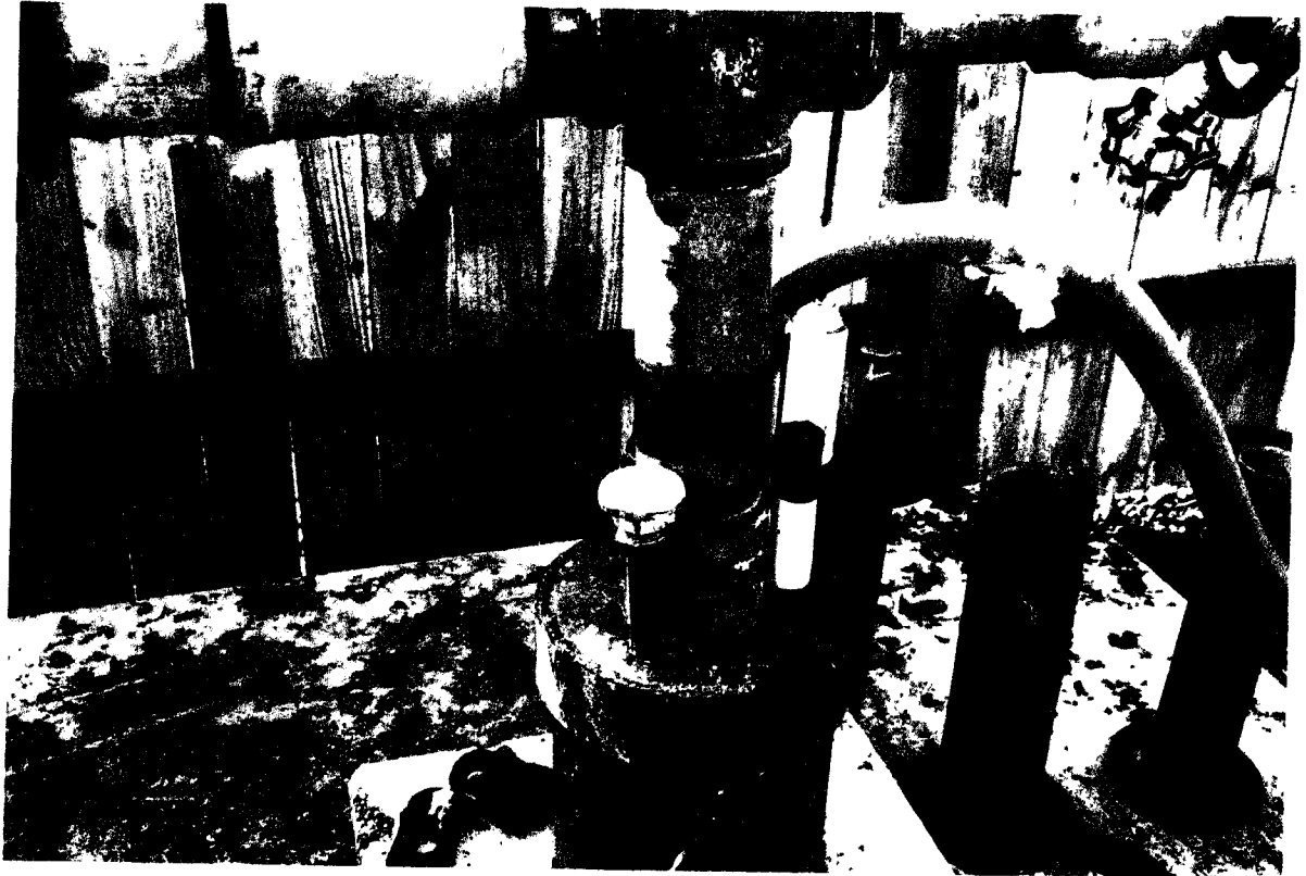
Screened Vent on Well Casing Well #3
