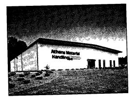
This shows a typical metal wall panel system available from most building system manufacturers. The panels come with a pre-finished baked enamel coating in a multitude of colors. Accessories such as doors, windows, vents, louvers, overhead doors, etc can be provided by the metal building manufacturer or purchased from commercial suppliers.
