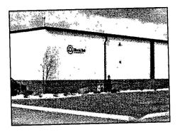
This photo shows a metal panel siding with a masonry wainscot. This option offers perhaps the best balance between initial construction cost, appearance, long-term maintenance, and durability. By using the more durable material, masonry, at the bottom of the wall, where most of the abuse is likely to occur, you protect the appearance of the metal panel/paint finish above. Given the reduced square footage of the masonry, the initial construction cost of the wall system can be controlled.
