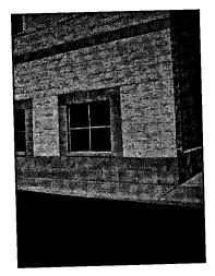
This photo shows a multi-color, multi-texture masonry veneer. Although this treatment can produce the most striking appearance, it comes at perhaps the highest per square foot cost of all options presented.
