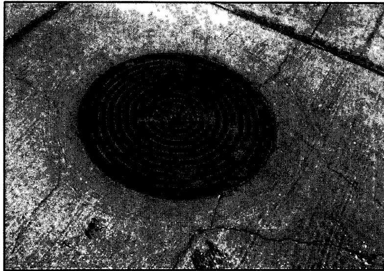
IMG_2227 SUGARBERRY PLACE SECTION 2 (COTTAGE GARDENS) - SANITARY SEWER MANHOLE LID
