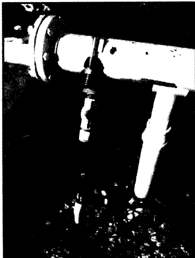
IMG_2223 PWS 1013271 - WELL NO 1 POLYPHOSPHATE CHEMICAL INJECTION POINT
