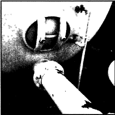
IMG_0925 PWS 1013271 - HPT MANWAY SIGHTGLASS AND DISTRIBUTION SYSTEM CONNECTION
