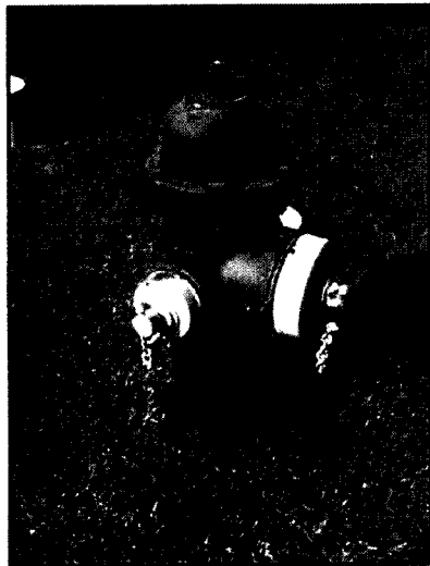
IMG_2230 PWS 1013271 - FIRE/FLUSHING HYDRANT
