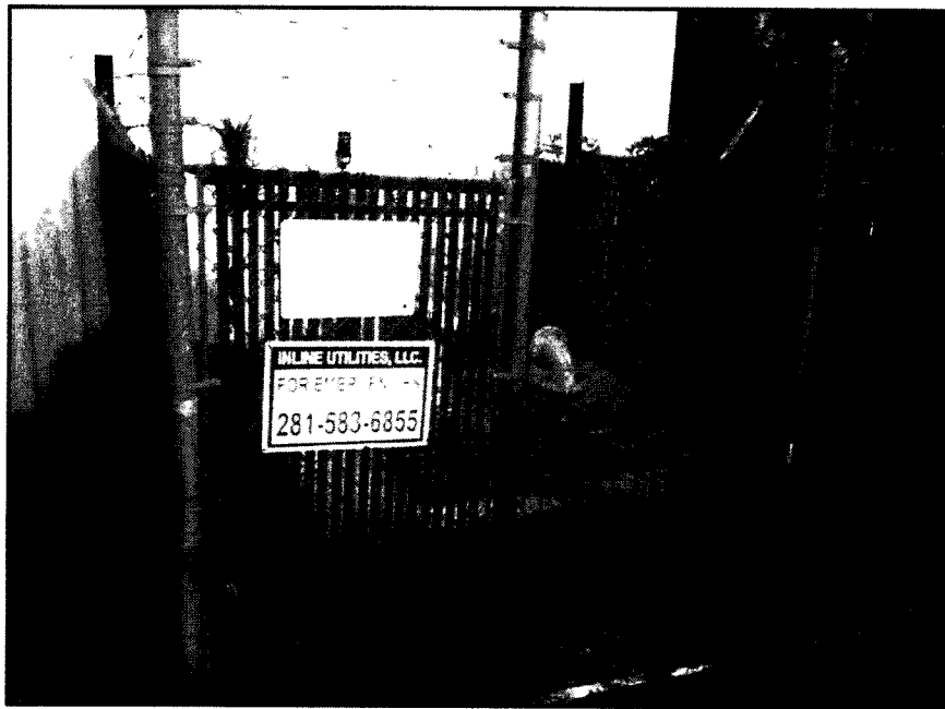
IMG_2174 SUGARBERRY PLACE SECTION 1 SANITARY SEWER LIFT STATION
