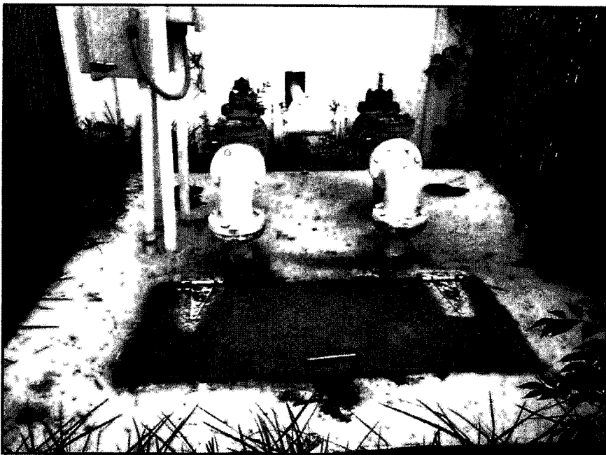
IMG_0864 SUGARBERRY PLACE SECTION 1 SANITARY SEWER LIFT STATION
