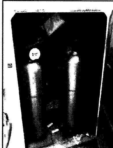
IMG_2182 WWTP - 150LB CHLORINE GAS CYLINDERS
