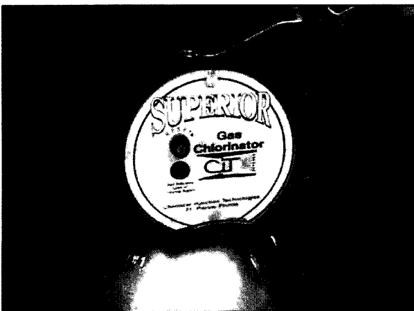
IMG_2183 WWTP - CHLORINE GAS CHLORINATOR
