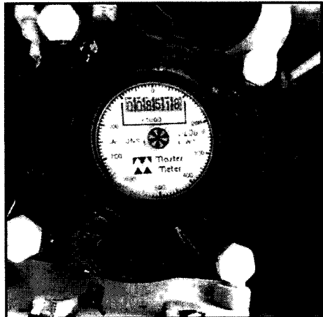
IMG_0929 PWS 1013271 - WELL NO. 2 TOTALIZING FLOW METER
