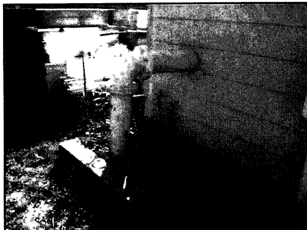
IMG_2225 PWS 1013271 - BOOSTER PUMP BUILDING DISCHARGE PIPING
