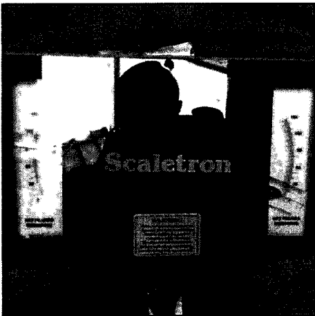
IMG_0911 PWS 1013271 CHLORINE GAS SCALE
