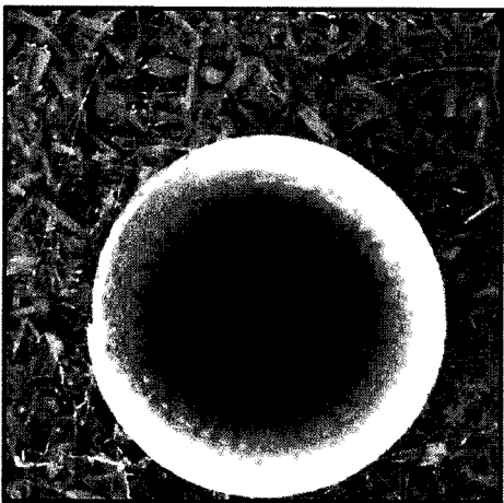
IMG_0948 PWS 1013271 - WATER DISTRIBUTION SHUTOFF VALVE BOX
