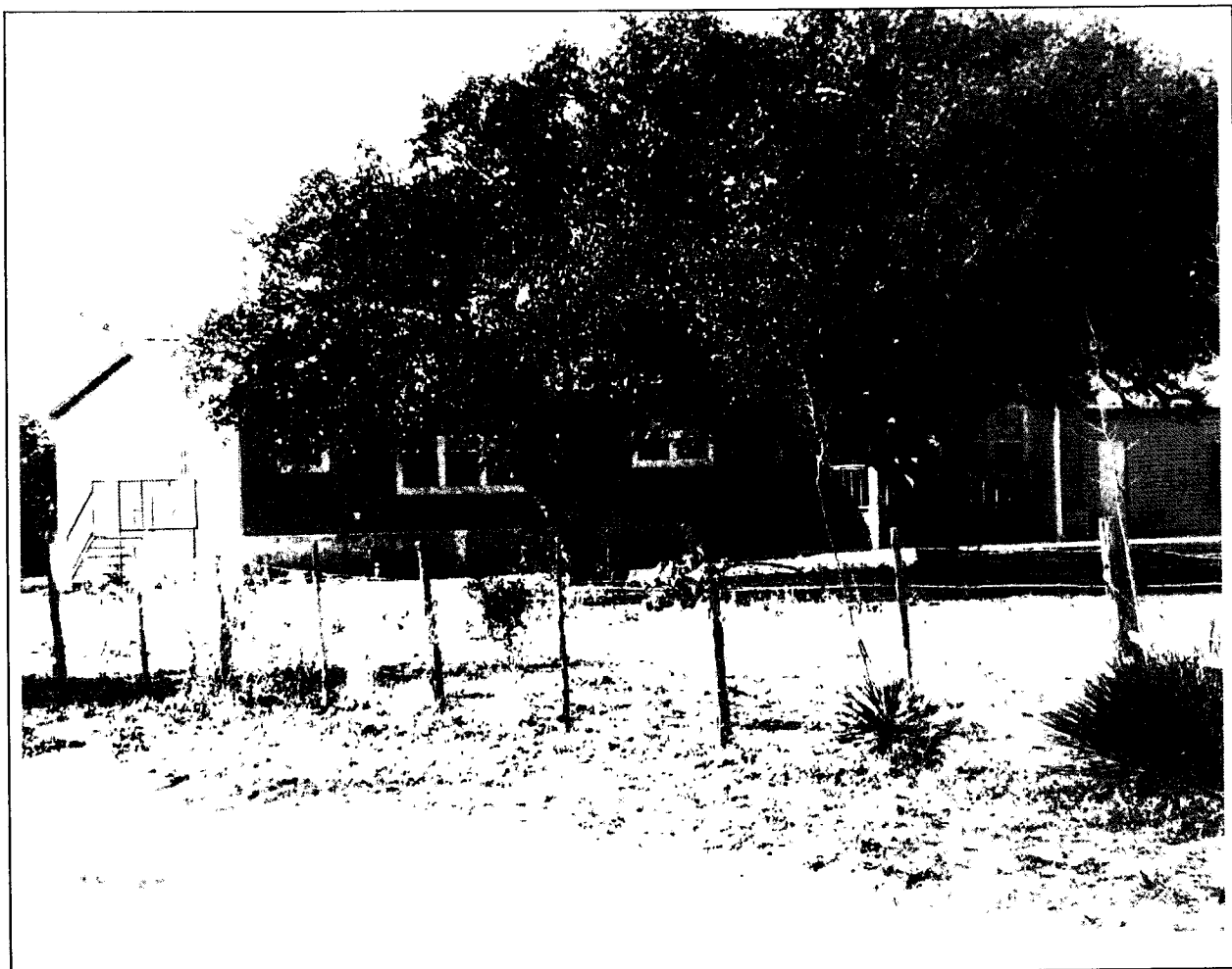
Habitable Structure 51 at 40 ft. N from ROW Centerline
