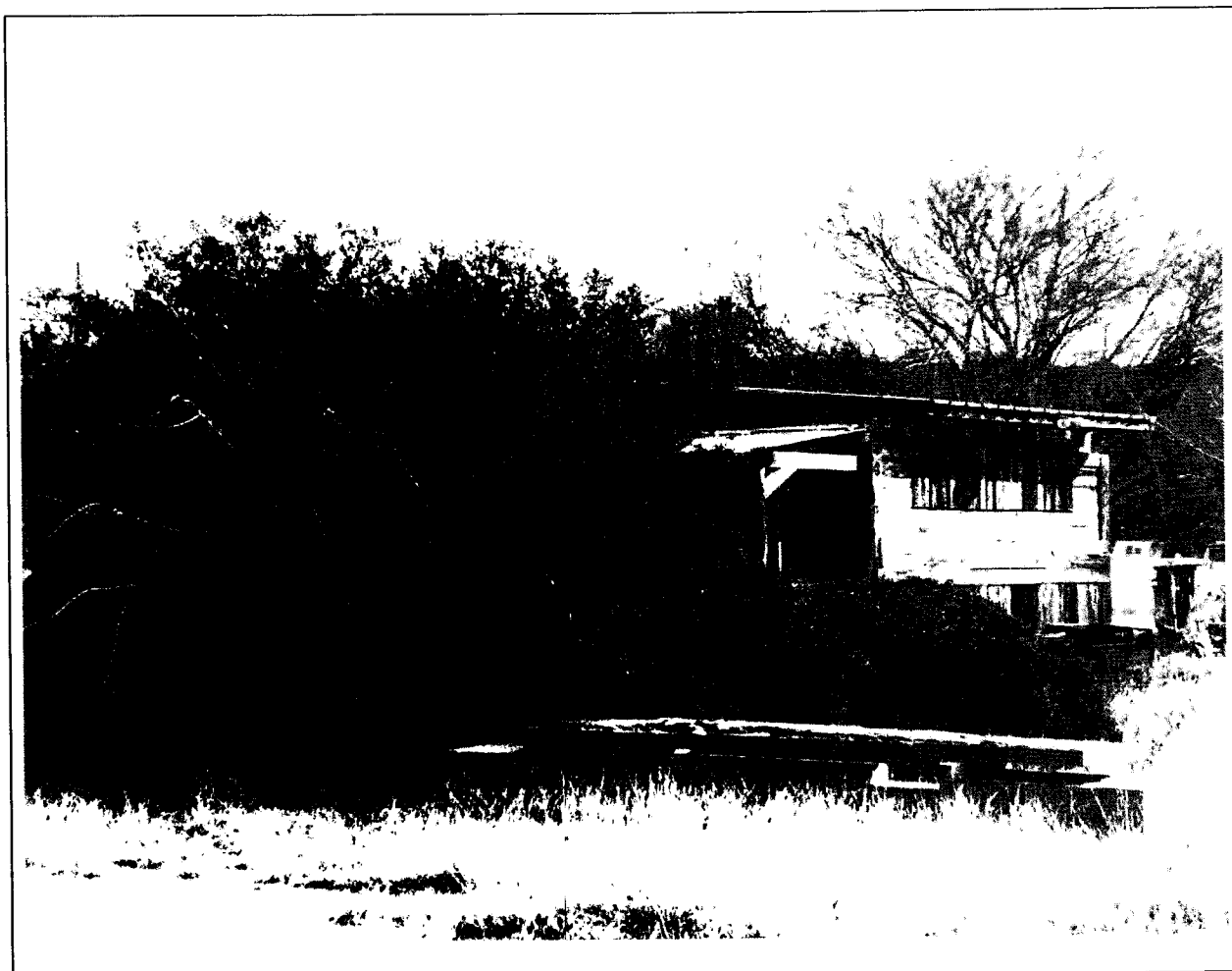
Habitable Structure 118 at 45 ft. N from ROW Centerline
